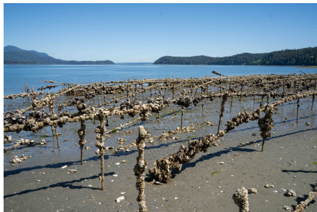
Derelict oyster farm structures near Harding Creek
